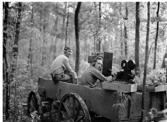
FIGURE 2. Paul Kellogg and J. J. Kuhn recording the Ivory-billed Woodpecker ( Campephilus principalis ) in Louisiana, April 1935, using the Cornell recording device.
