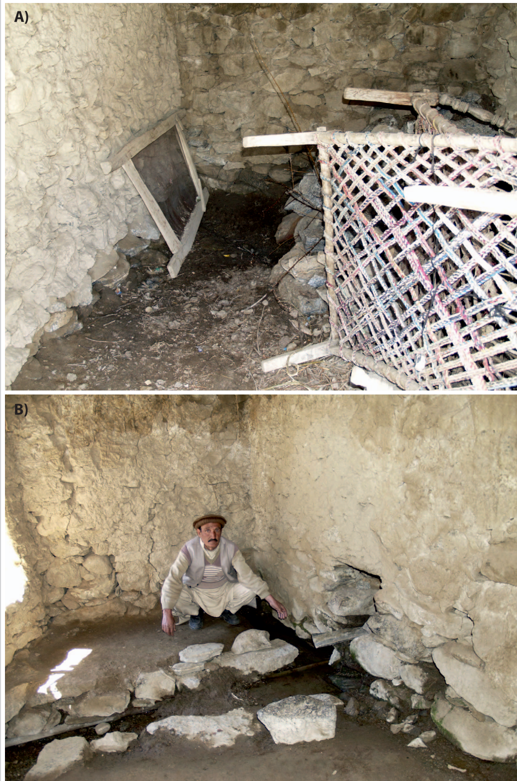
FIGURE 3 (A) Seepage inside a house located below an irrigation channel; (B) cracks in a house as a result of heavy seepage. (Photo A by Jawad Ali; photo B by Muhammad Asad Salim)
