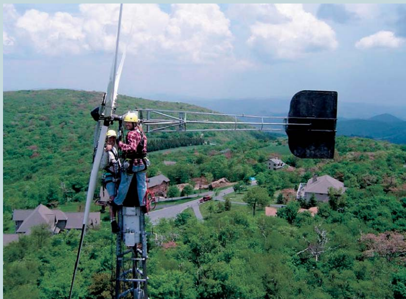
FIGURE 4 Students replace blades at Beech Mountain research site. (Photo courtesy of ASU Small Wind Initiative)
